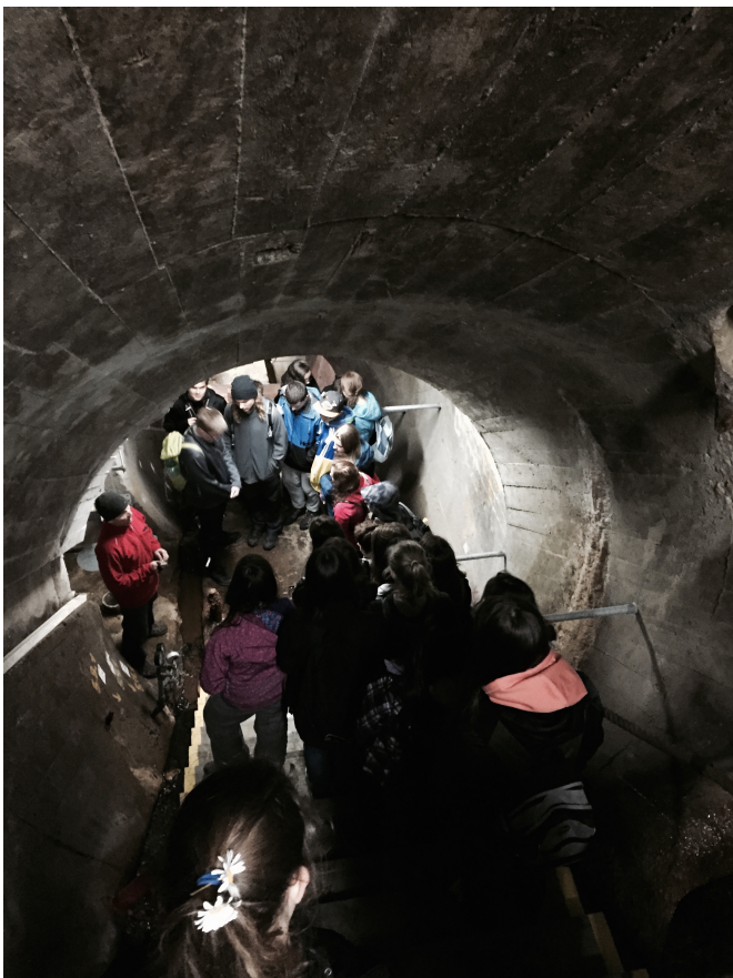
Pictures: inside of the dam, Hydroelectric dam Vír I.
